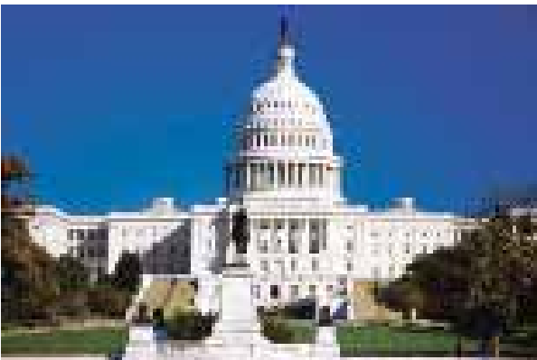
U.S. Capitol Building, Washington, DC
